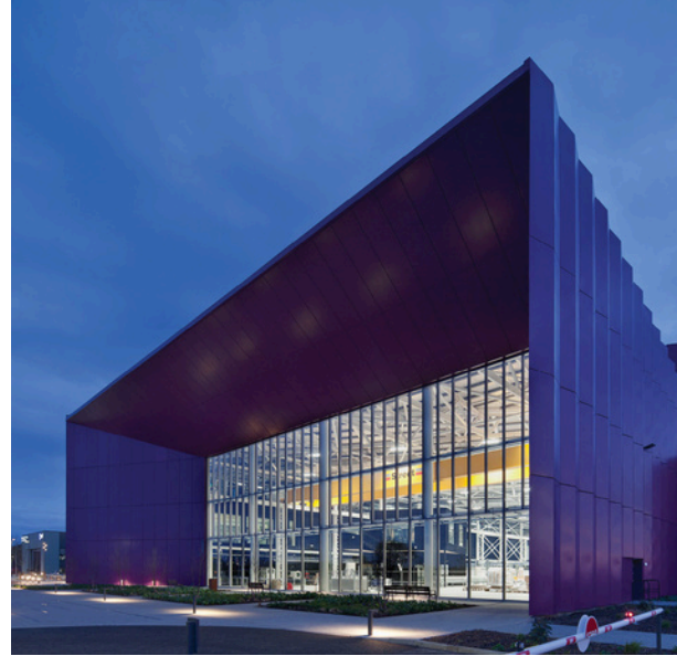
The NMIS Netherton building is designed to be carbon neutral. Image: David Barbour Photography
