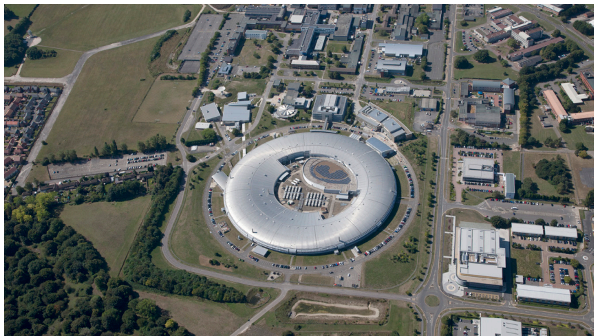
RAL is located on the Harwell Campus (aerial view).
